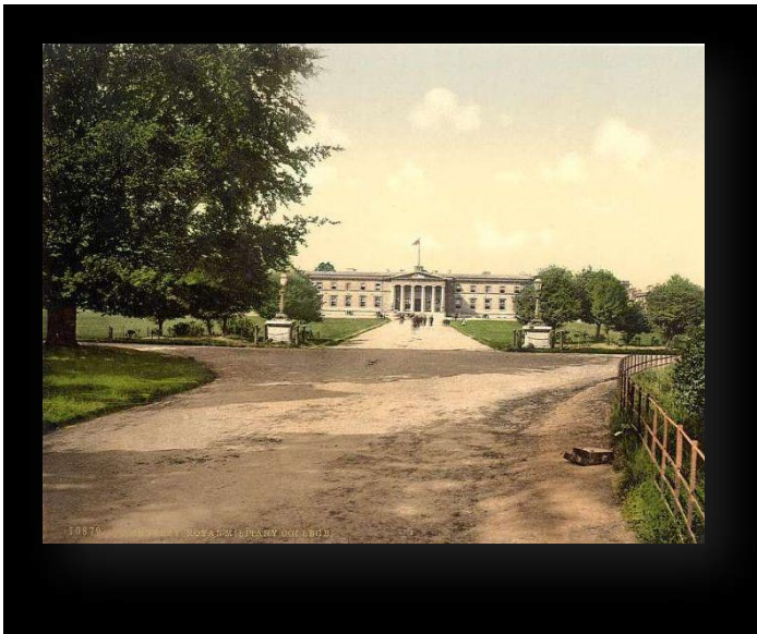
Sandhurst, main building, ca. 1900
